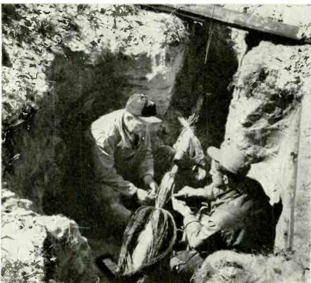
Courtesy Bell Telephone Cable splicer and helper installing buried cable.
